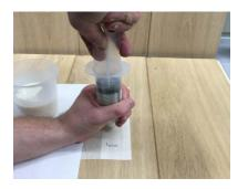
7. Press mixture into the hollow spot. Continue until hollow spot is entirely filled. Weigh down filled areas for approx. 2 h, if necessary
